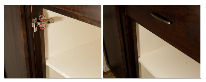
Remove the screws that go into the cabinet frame from the hinge, then remove the hinge.
