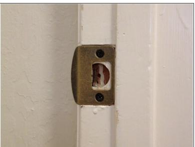
Place the strike plate back on the door frame and tighten the screws.
