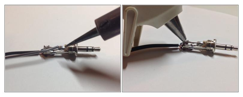
• Solder over each lead's hole, connecting the wire to the lead.
