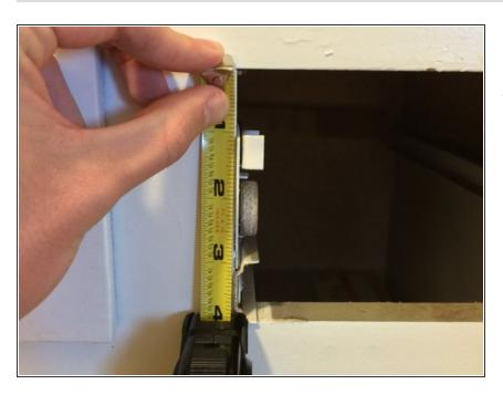
Make sure the height of the wheel tracks matches up with the height of the guide tracks by measuring down from a shared point between the drawer and cabinet.
