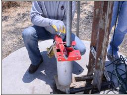
Once the riser main has reached the block and tackle, tighten the base clamp against the riser main.
