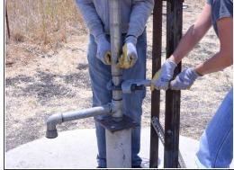
Use a pipe wrench to fully loosen the above grade riser pipe.
