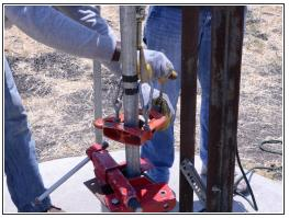
Remove the clamp from the riser main, and repeat steps 23-25 until first joint is exposed.
