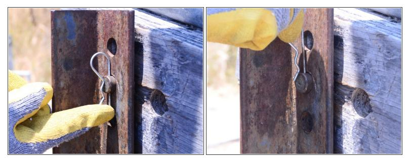
• Lift the two pins attaching the pump frame to the head and handle up, off of the pump frame.
