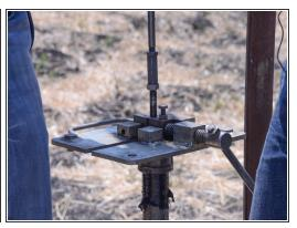
Attach and tighten the rod clamp a few inches below the first pump rod connection.
