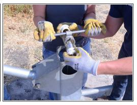
• While one person lifts up on the T-handle, remove the bolt and connection pieces.
