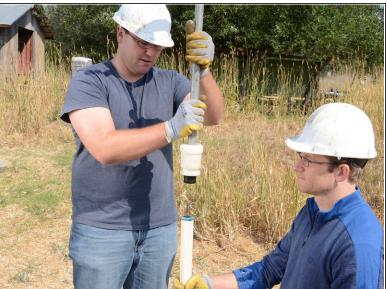
• Lift and remove the handle from the pump. Store the handle in a sanitary place to prevent contamination.
