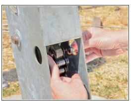
Remove the nut from the chain bolt.
