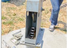
Pull the top of the chain straight off of the pump handle.
