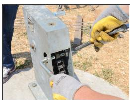
Using the two access holes, place an angled socket wrench on the bolt and nut attaching the chain to the pump handle.
