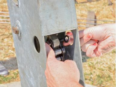
Remove the washer from the chain bolt.
