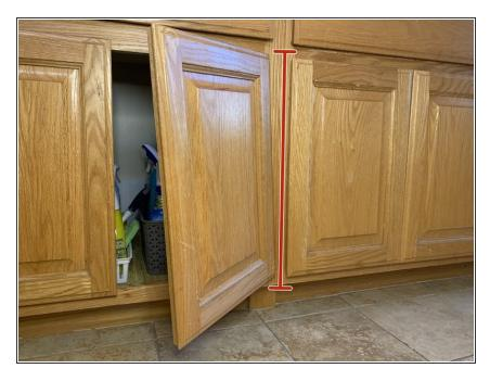
Open the cabinet door, and determine where it is misaligned.
