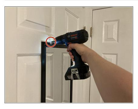
Replace the top brackets and tighten them to full secure the mirror.
