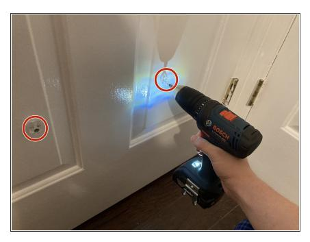
Loosen, but don't remove, the bottom brackets to accommodate the width of the new mirror.
