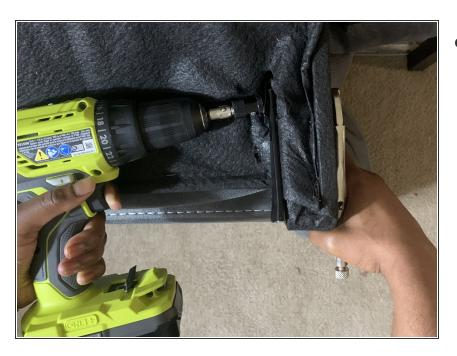
Use a drill and vice grips to secure the bolt on the screw.
