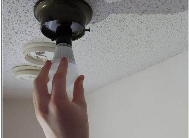
Re-screw the lightbulb into the fixture.
