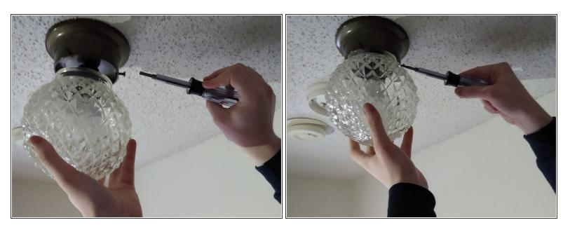
Hold onto the fixture, and screw it back in with the screwdriver.
