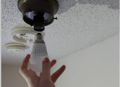
Unscrew the lightbulb from the fixture.
