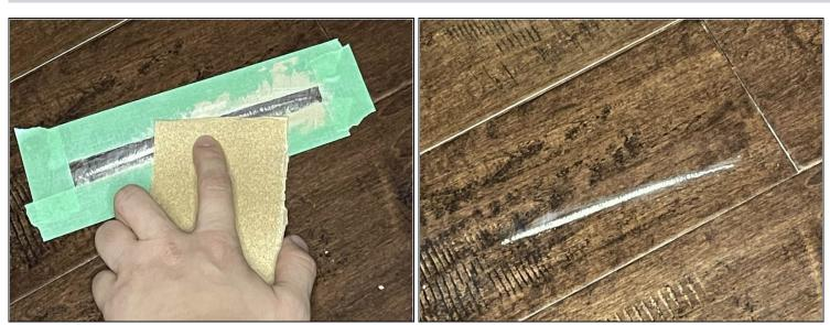
• After drying for 10-15 minutes, sand the area down until the wood filler is level with the rest of the floor.
