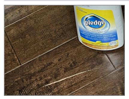
Using a hardwood cleaner and a clean cloth, wipe the area down to remove any dirt or debris.
