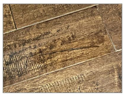
After applying the wipe on polyurethane, your scratch should now be blended in with the rest of the floor.
