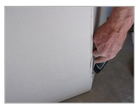
Use your utility knife to cut the new piece of wallboard, making it a little smaller than the actual size of the ceiling opening, so that the installed piece will have a small gap around the edges.
