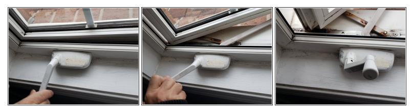
Turn the window handle clockwise to open the window.
