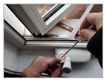
Use a flathead screwdriver in a clockwise direction to remove the 2.11 mm screw from the bottom of the window handle.
