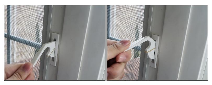
Unlock the window lock by flipping both switches up until they are pointed horizontally outwards, facing the user.
