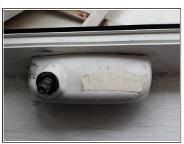
• Turn the loosened window handle in either direction to remove it.
