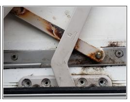
• Using a Square #0 screwdriver, remove the four 25.4 mm screws placed on the outside of the window sill.
