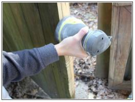
Sand the edge of the gate that was cut using a power sander until the edge is smooth and fits properly when closing the gate.
