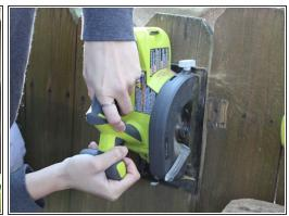
Starting at the bottom of the gate, place the power saw on the sharpie line and cut along the entirety of the line.
