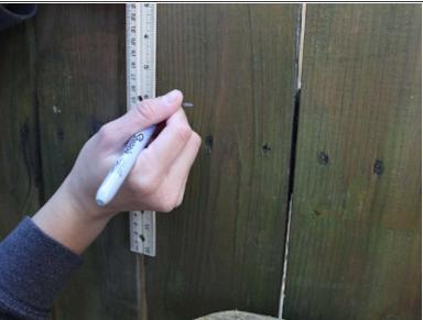
Using a ruler, measure 6 inches down from the top of the gate and mark that spot using a sharpie.
