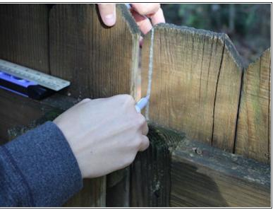
Using a ruler and a sharpie, draw a line starting at the bottom corner of the gate to the top corner
