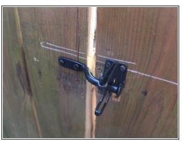
On the adjacent fence at the marked spot attach the second half of the latching mechanism using a power drill and screws.
