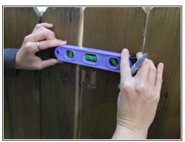
Using a ruler, measure 6 inches down from the top of the adjacent fence and mark the spot using a sharpie
