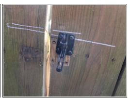
At the marked location on the gate, attach the latch for the gate using a power drill and screws.
