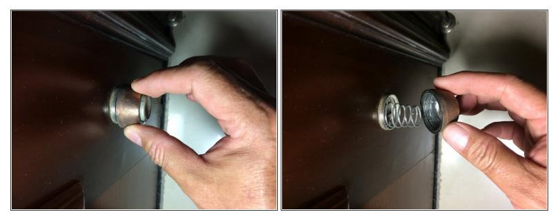
• Remove the old door fitting by rotating it counter-clockwise.
