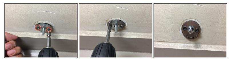
• Using a screwdriver or a drill, attach the new mount base to the wall with the two screws.
