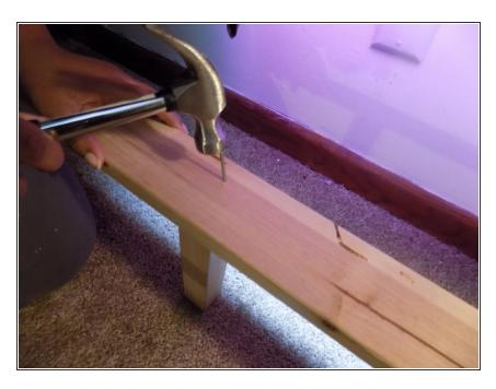
Hammer the 50 mm nails down into the slat and into the wooden plank.
