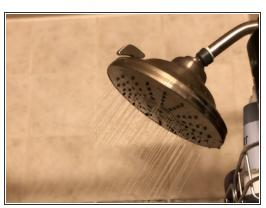
Twist the shower head back onto the pipe and tighten it with the pipe wrench.
