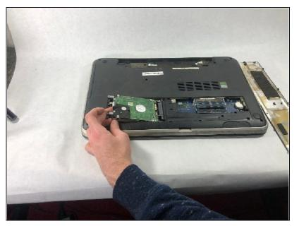
Grabbing from the left of the hard drive, slide the part to the left and pull up, lifting it away from the machine.
