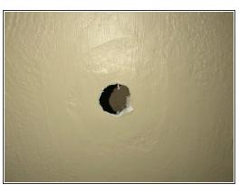
• Use pliers (or tweezers if the hole is very small) to clean out hole by removing the drywall out of the hole.
