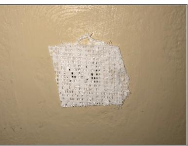
Use a damp sponge to apply moisture to make the mesh stick to the wall, covering the entire hole.
